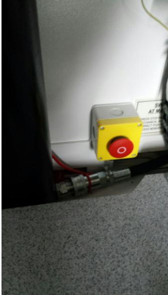
Photo of the rerouted hose
